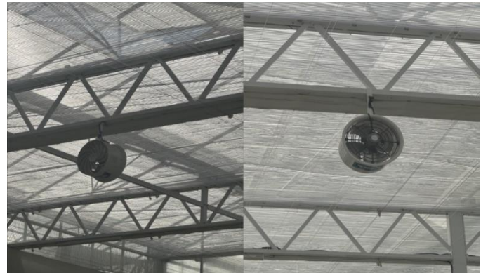
Figure 2 Circulation ventilation fan installed in the semi-enclosed greenhouse under study
