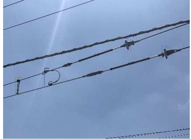
Fig.7 Overhead line detection
