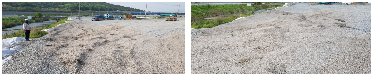
Fig. 1. Ground deformation according to construction of GCP method
